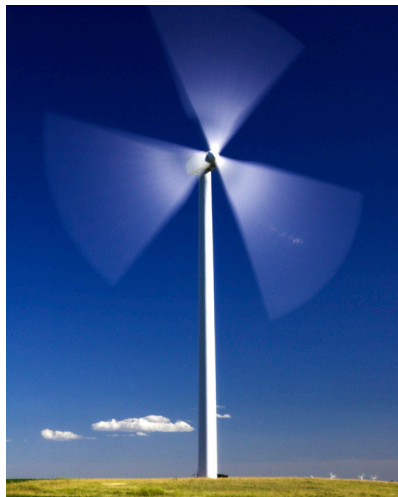
The average rotor diameter has increased from 75 meters in 2005 to 102 meters in 2015, according to the American Wind Energy Association. (Courtesy: Logisticus Project Group, LLC)
